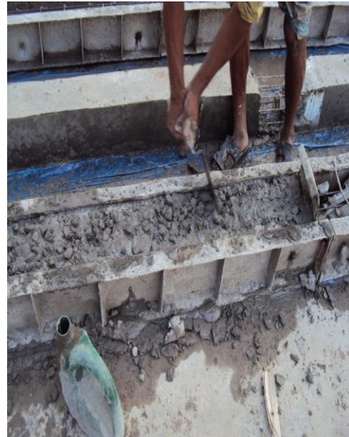
Fig. 2.43 Casting of concrete (step 05)
