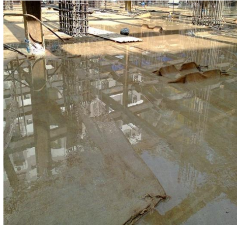
Fig. 2.33 Concrete curing
