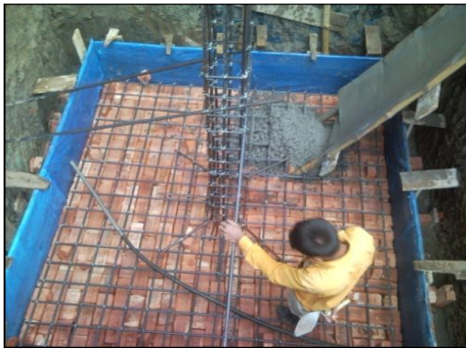
Fig. 2.16 Casting of concrete (step 08)
