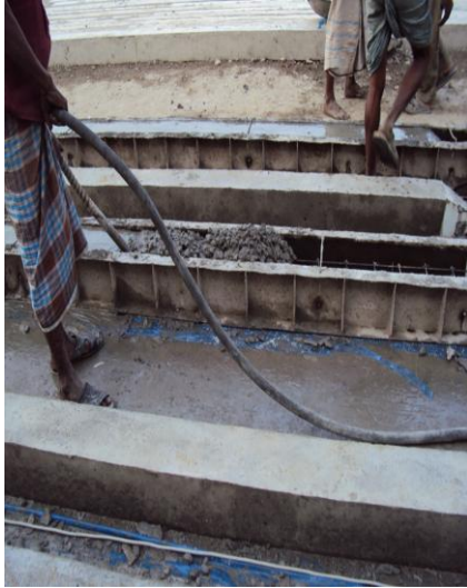
Fig. 2.44 Compaction of concrete (step 06)
