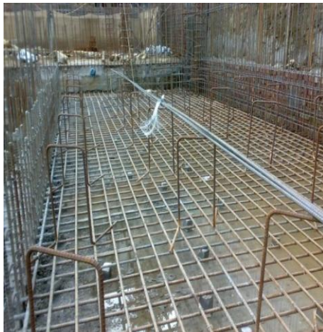
Fig. 2.31 Reinforcement placing (Bottom mesh)
