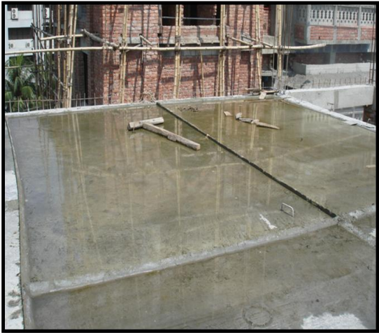
Fig. 3.33 Ponding
