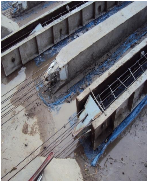
Fig. 2.42 Inserting steel cap (step 04)
