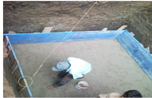
Fig. 2.11 Leveling and dressing (step 02)
