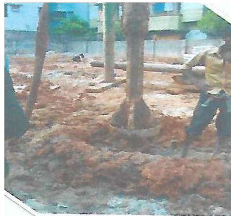
Fig. 2.48 Centering and Placing of Auger
