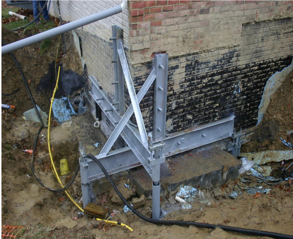
Fig. 7.2 Underpinning
