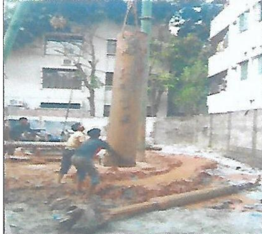
Fig. 2.49 Temporary Casing insertion
