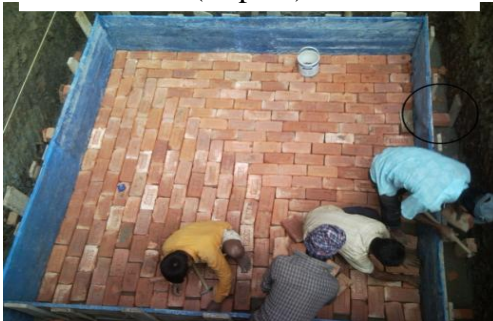
Fig. 2.12 Brick flat soling placement (step 03)
