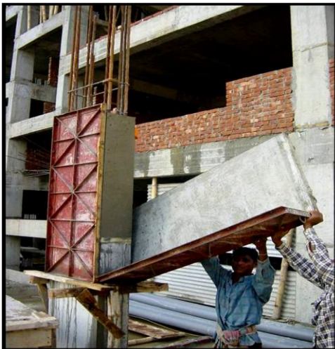
Fig. 3.12 Removal of shuttering
