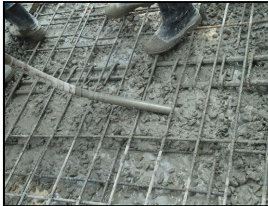
Fig. 3.31 Compaction
