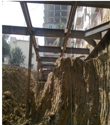
Fig. 2.23 Strutting and bracing
