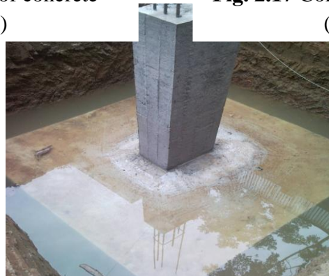
Fig. 2.18 Curing of concrete (step 11)
