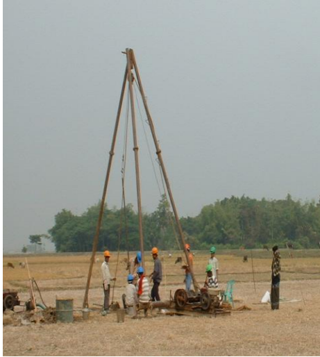
Fig. 2.3 Placement of pipe derrick (step 01)
