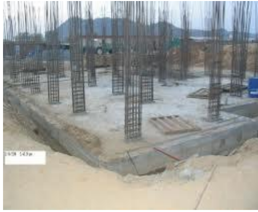
Fig. 2.20 Mat foundation
