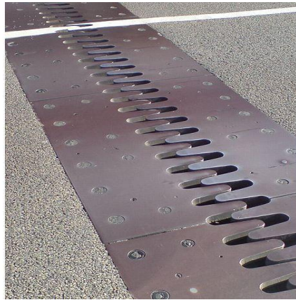
Fig. 6.2 Expansion Joint
