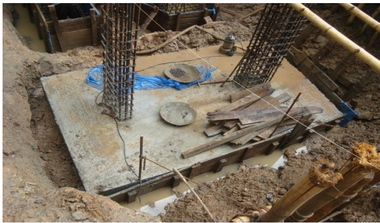
Fig. 2.19 Combined foundation
