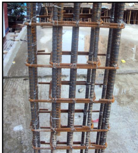
Fig. 3.3 Ties of column
