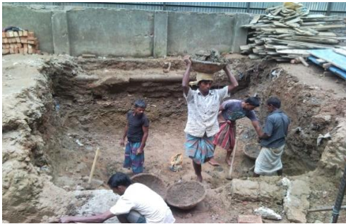
Fig. 2.10 Excavation of trench (step 01)
