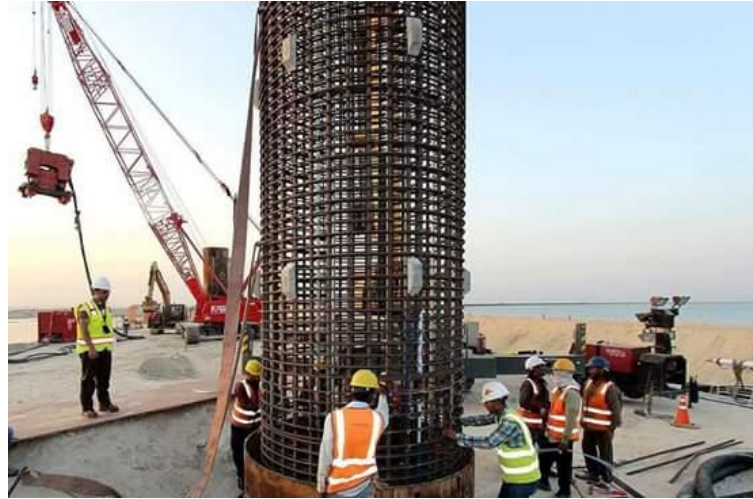
Fig. 2.53 Welding of casings
