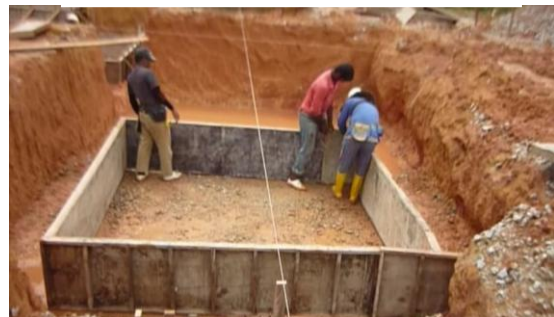
Fig. 2.13 Shuttering placement (step 05)
