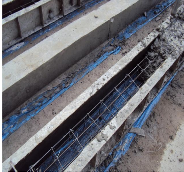
Fig. 2.41 Placing of shuttering (step 03)
