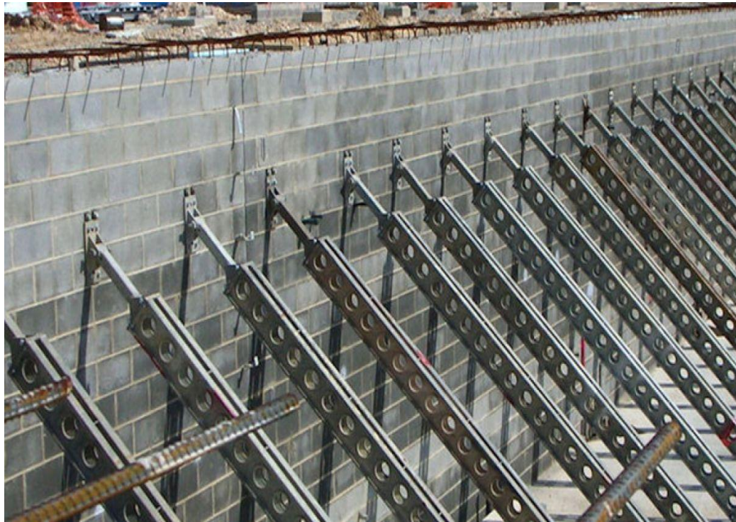
Fig. 7.1 Structural Shoring
