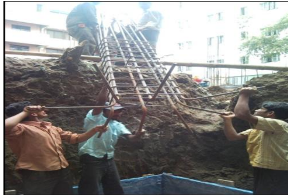
Fig. 2.15 reinforcement placement (step 07)
