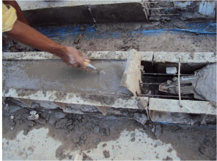
Fig. 2.45 Leveling top surface (step 07)
