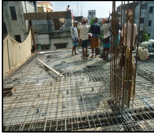
Fig. 3.30 Concrete casting
