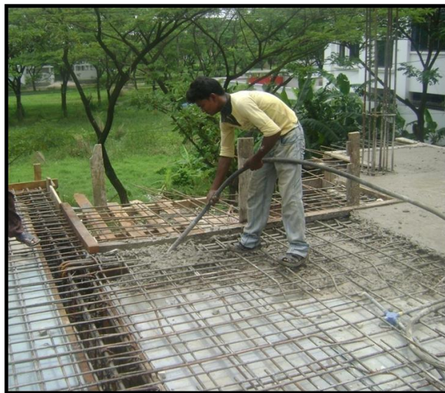
Fig. 3.23 Monolithic casting of beam and slab
