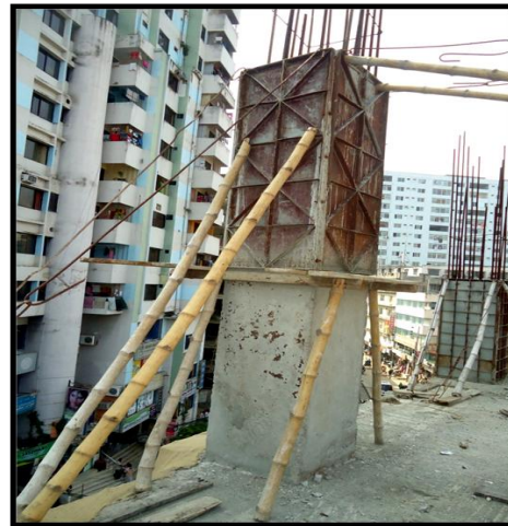
Fig. 3.10 Concrete Casting in two lifts
