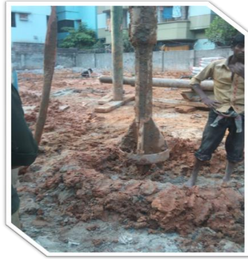
Fig. 2.4 Centering and Placing of Augur (step 02)
