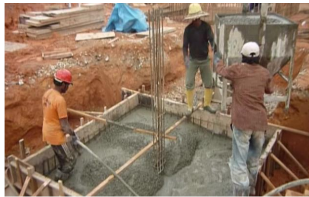
Fig. 2.17 Compaction of concrete (step 09)
