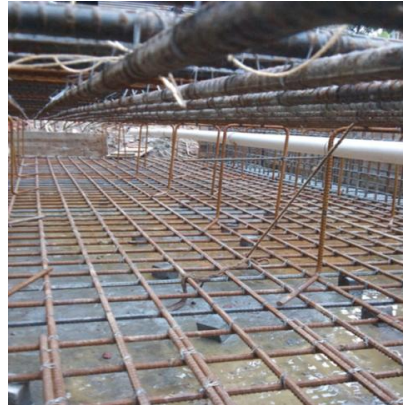
Fig. 2.30 Placing CC block
