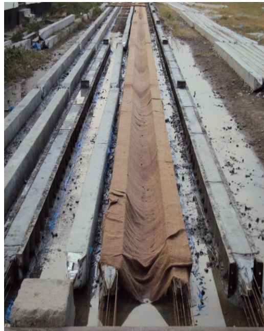
Fig. 2.46 Curing of concrete (step 08)
