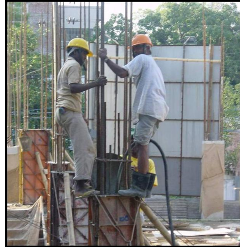
Fig. 3.9 Use of vibrator
