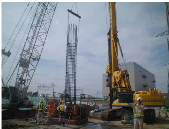
Fig. 2.52 Reinforcement casing placing
