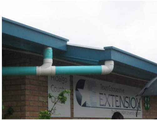
Fig. 8.2 Rain Water Spout
