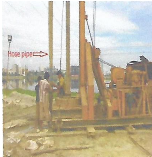
Fig. 2.50 Provision for hose pipe
