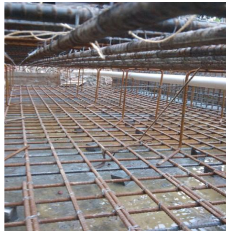
Fig. 2.32 Reinforcement placing (Top mesh)
