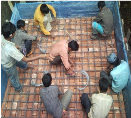
Fig. 2.15 reinforcement placement (step 07)
