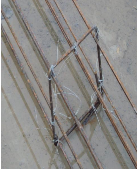
Fig. 2.40 Reinforcement casing construction (step 01)
