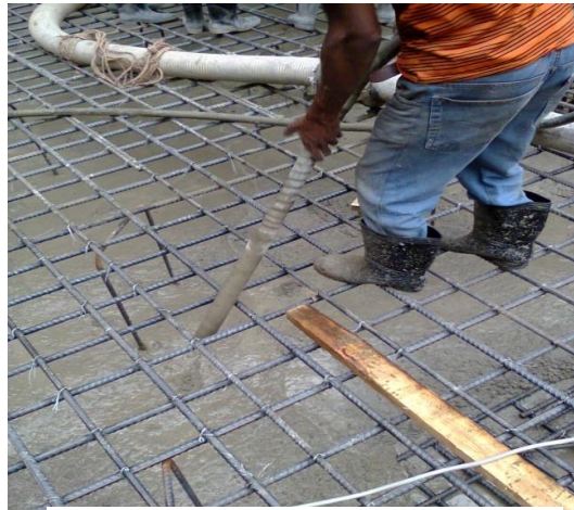
Fig. 2.34 Concrete compaction
