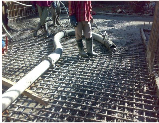
Fig. 2.33 Concrete casting
