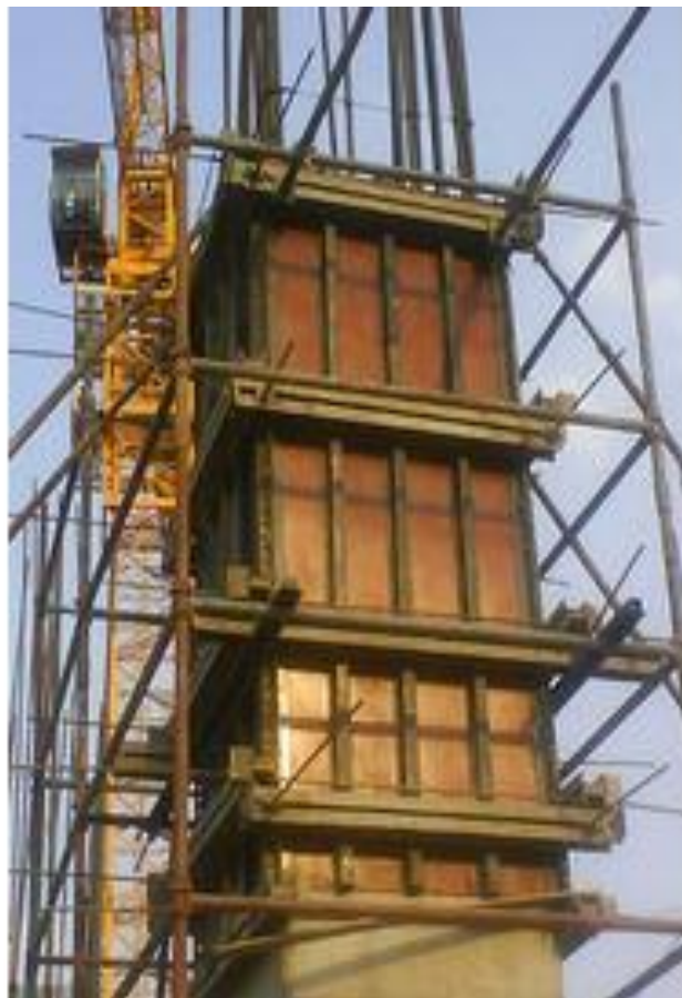
Fig. 11.1 Shuttering
