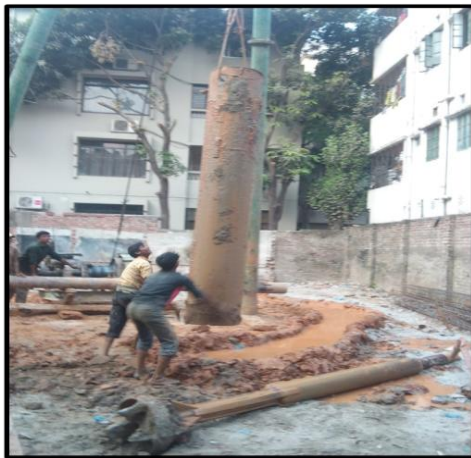
Fig. 2.5 Temporary casing placement (step 03)
