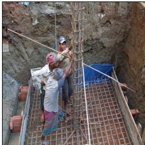
Fig. 3.1 Placing column reinforcement
