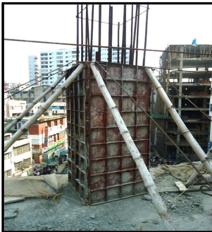
Fig. 3.10 Concrete Casting in two lifts
