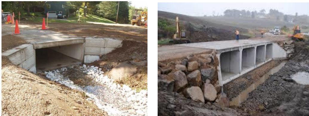
Figure 4.4: Box Culverts ( http://www.hudsoncivil.com.au )
