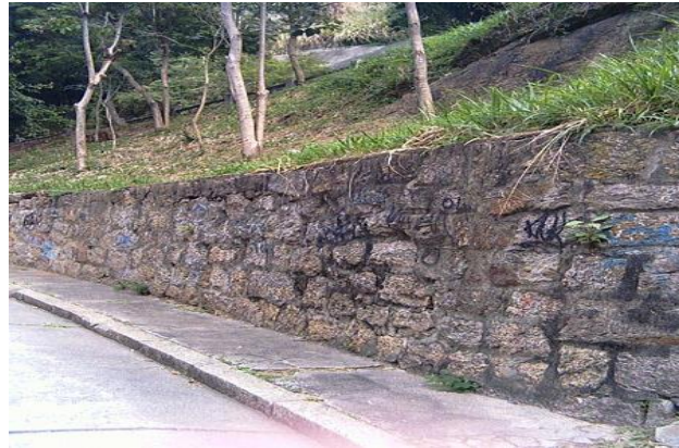
Figure 6.1: Typical Retaining wall
