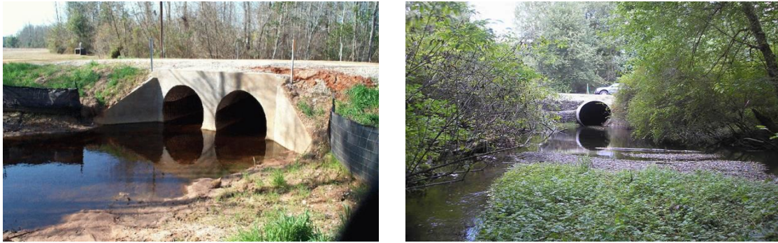
Figure 4.3: Pipe Culverts ( https://www.civilgeo.com )
