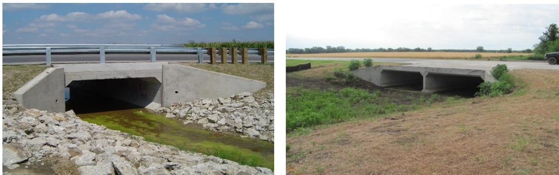
Figure 4.3: Slab Culverts ( http://www.lefiltredumonde.com )
