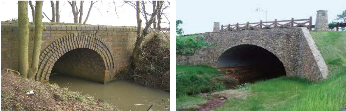
Figure 4.2: Arch Culverts ( http://www.conteches.com , https://qph.ec.quoracdn.net )
