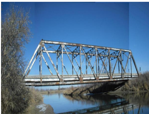
Figure 1.2(a): Truss bridge (Trenton through truss bridge, 2008)
