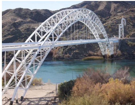
Figure 1.2(b): Arc bridge (Old trails arch bridge, n.d.)
