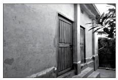
Figure-13: High plinth in the newly constructed buildings. (Source: Author's photographs)
